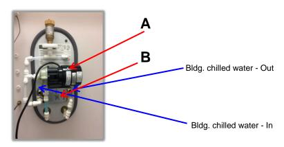
**C.** Measured Flow Rate of Ecodenser (unrestricted from output orifice): .92 gal/minute. <u>Output</u> water valve: .21" dia.
